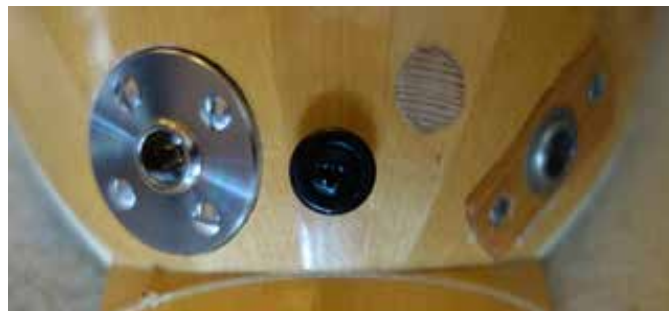
Jacks and a strap holder fitted to the front block.
